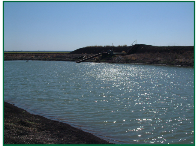
A storage cell
